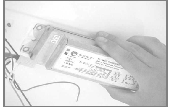
Mounting NU III ballast onto a lighting fixture.
